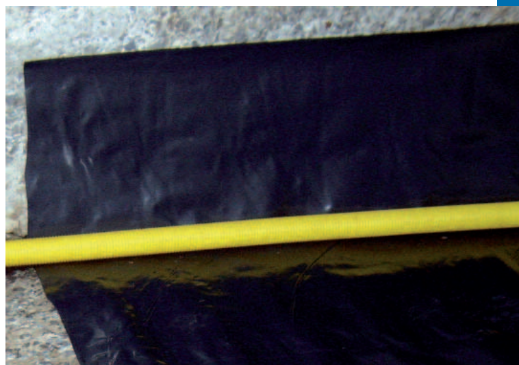
Photo 4: Protecting silage pit wall-floor joints
