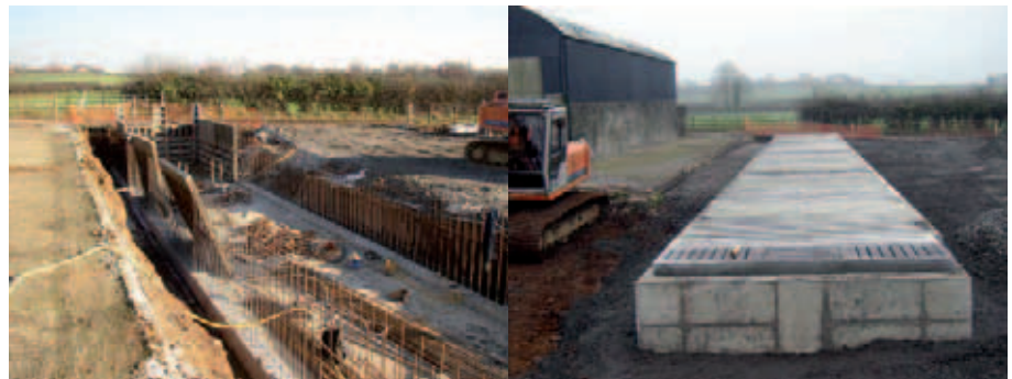
Photo 6 Left: Slurry tank under construction. Right: Slurry tank completed.
